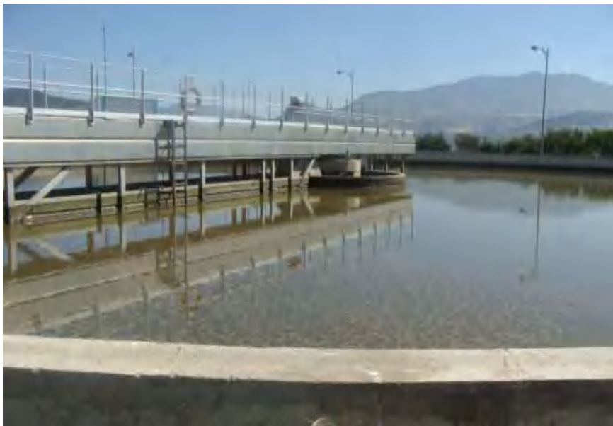
Figure 16: Clarificateur de la station de Sidi Merouane.
