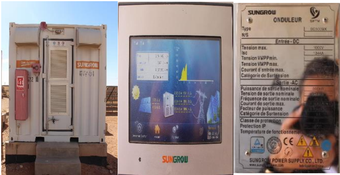
Fig.4.9 SUNGROW Inverter (Shelter)
