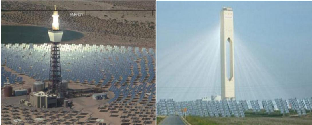
**Figure I-17:** Receveur central solaire Barstow, California
