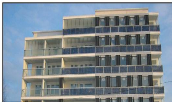
Fig.III.15. Garde-corps de balcon.
